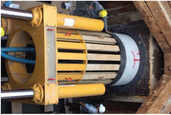
Figure 4. Pipejacking a pipeline D1500mm cross Nguyen Van Linh road, Binh Chanh district, Hochiminh city (Baogiaothong, 2018)
